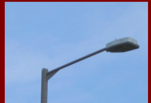
High pressure sodium (SON) Full Horizontal Cutoff (FCO /HCO)
