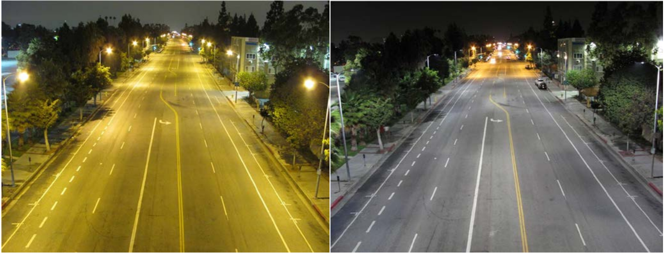
Figure 4 Absence of uplight from modern luminaires at right compared to older drop-lens fixtures at left. (Photo credit: LABSL)
