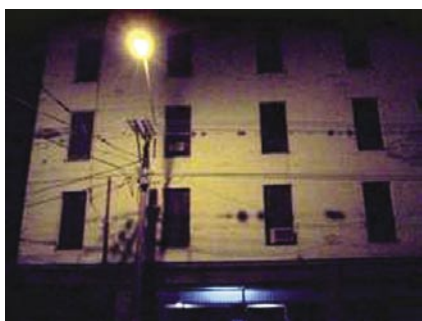
Figure 3. Facade before retrofitting
