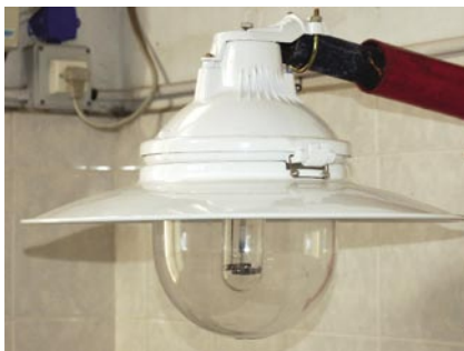
Figure 2.- Luminarie after retrofitting.
