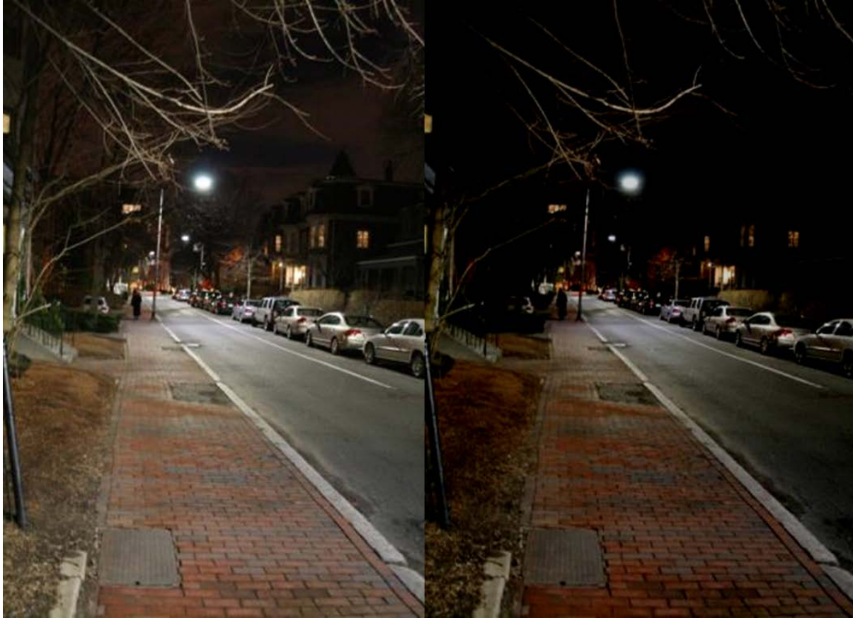
Figure 8. 4000 K LED Street Lighting System in Cambridge, MA, shown at initial startup at dusk (left) and 50% dimmed after midnight (right). Photos: WSP | Parsons Brinckerhoff
